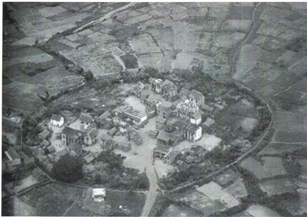
The buildings of walls in an effort of protection.
